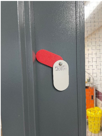
Door flag showing two colours shows that the room needs to be evacuated.
